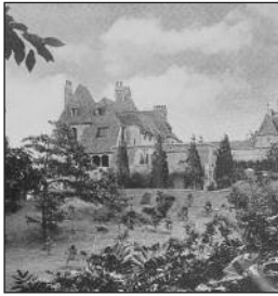
Built for Daniel Guggenheim's son, Harry Guggenheim, Falaise was constructed in 1923 to the design of Frederick J. Sterner, architect. Built in the style of a French Norman manor house, the siting of the house overlooking water explains the name "Falaise", from French for cliff.
